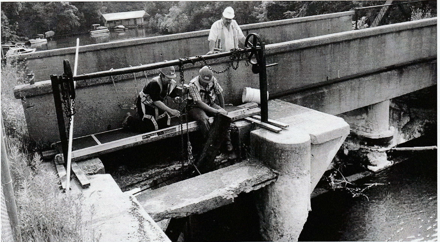
Two workers under the direction of a Norfolk County foreman removed the first stop log Tuesday morning at Misner Dam.
