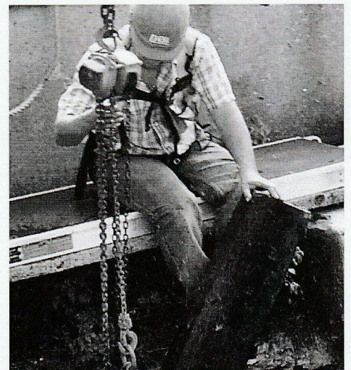
A worker uses a hoist to pull the first of the unauthorized stop log from the sluiceway at Misner Dam. The log was later expected to be cut into pieces.
